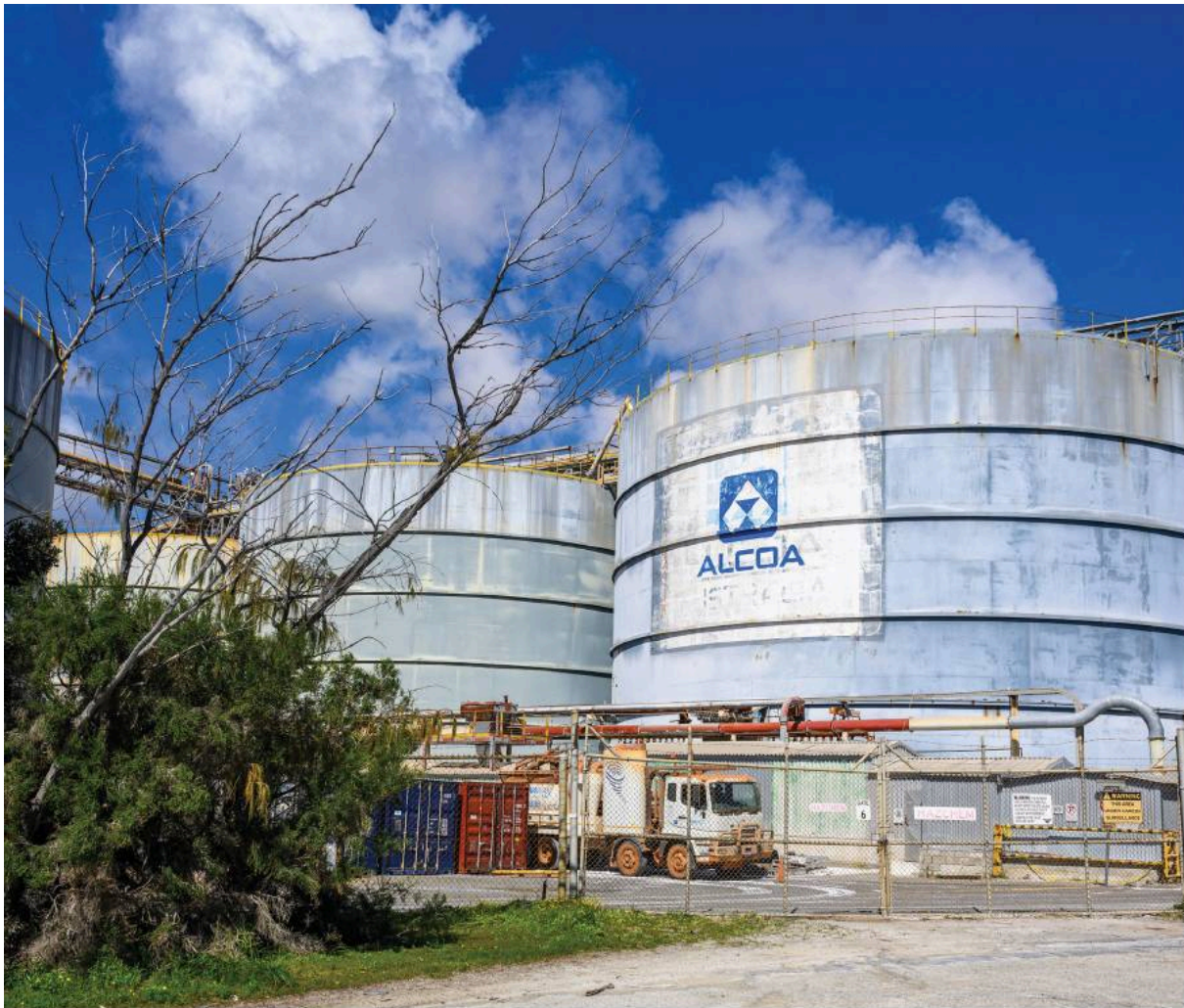
Alcoa completed shutdown of its Kwinana alumina refinery on schedule in June. Photo: David Henry
